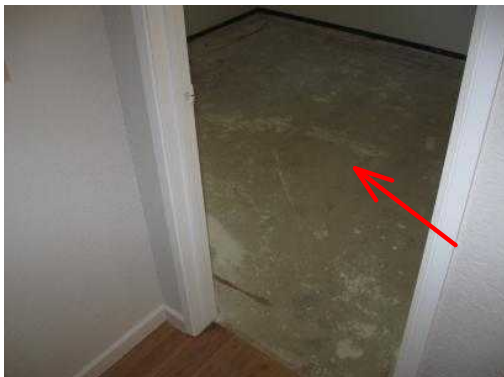
Missing right/front bedroom area flooring noted. Cracking noted at the slab.
