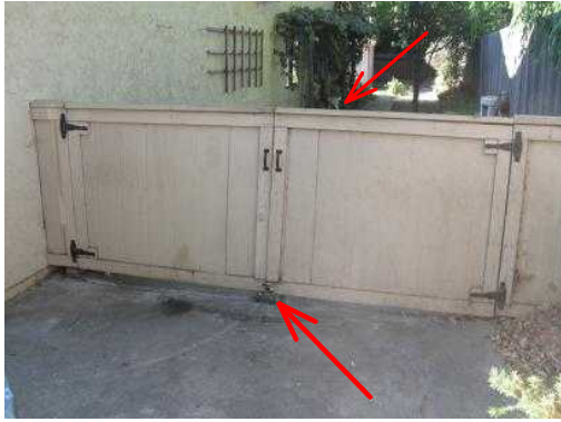
The right side gate is damaged and deteriorated. There is a pad lock on the right side gate.
