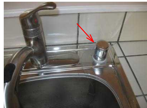
Dishwasher drains thru air gap. Clean drain line and re-test. Consult a licensed plumber.
