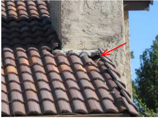
Slipped down rear roof tile noted, at base area of chimney. Repair, as required.
