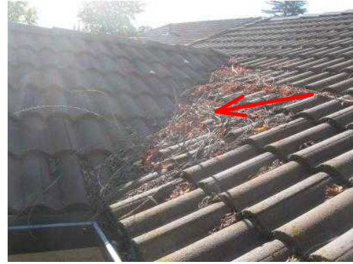
Debris located in metal valleys. Recommend cleaning the valley areas, for proper roof drainage.
