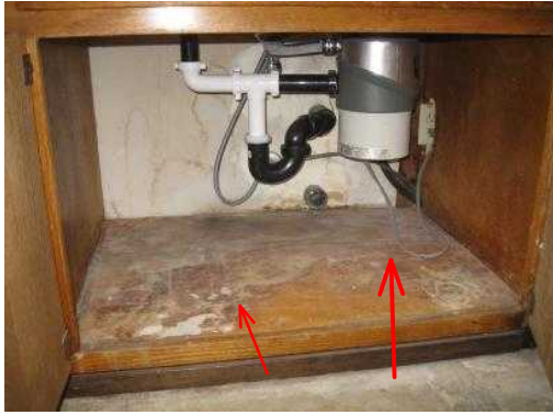
Evidence of prior leakage. Stain in kitchen sink base cabinet bottom. See pest report.
