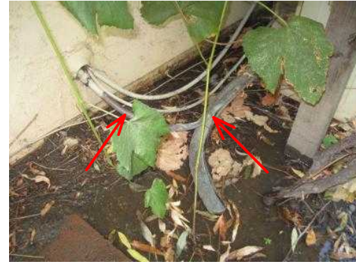
Missing insulation, at the low/high pressure lines. Replace insulation, as required.
