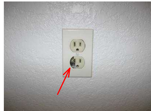
Broken right side/middle bedroom right side wall outlet. Consult a licensed electrician for repairs.
