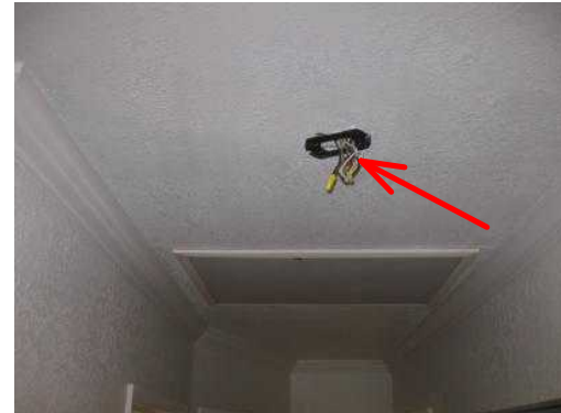
Missing hallway ceiling smoke detector unit noted. Replace, as required.
