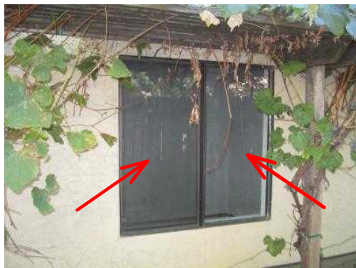
Failed seal noted at right side/middle bedroom window. Repair, as necessary.
