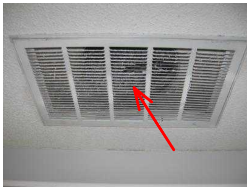
The filter is missing, at the master bedroom walk-in closet area ceiling cold-air return.
