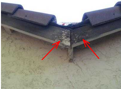
Wood deterioration noted to fascia/barge rafter, at right side of house, at the valley area.
