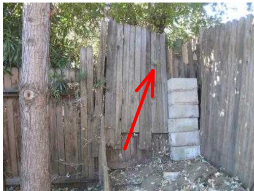
Right/rear fence section is broken/damaged. Repair/replace fence sections, as necessary.
