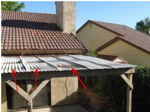
Loose/bent top patio cover fiberglass panels noted. Repair, as necessary.
