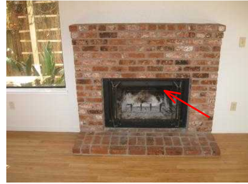
Creosote build-up noted. Have cleaned and liner re-checked, prior to use.
