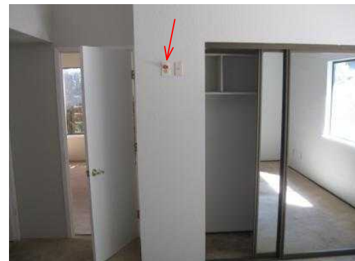
Reversed polarity, at master bedroom upper wall outlet, next to the bypass closet doors.
