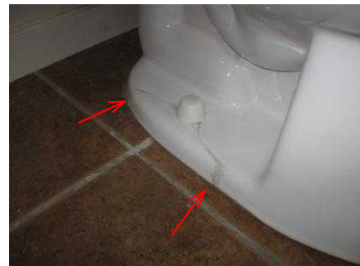
Crack noted at the left side base of hall bathroom toilet. Recommend replacing the toilet.
