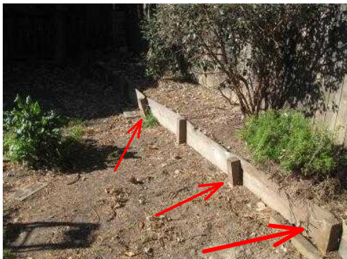
Wood timber retaining wall at right side is leaning and posts are deteriorated.
