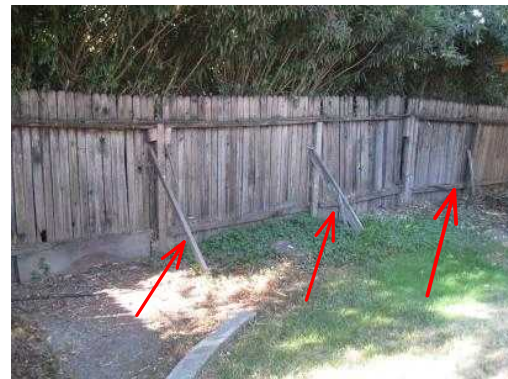
Rear fence sections are being held up by boards. Repair, as required.
