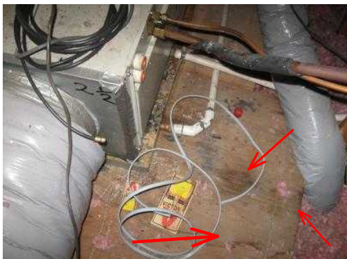
Water stains noted at the plywood base, under the heating unit in the attic. The area was dry, at the time of inspection. Refer to seller for disclosure.
