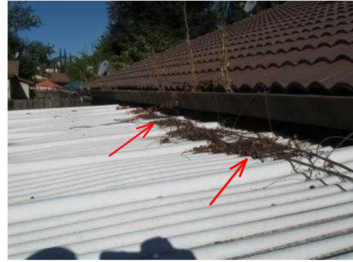
Debris on patio roof. Keep clean, to assist in preventing damage.
