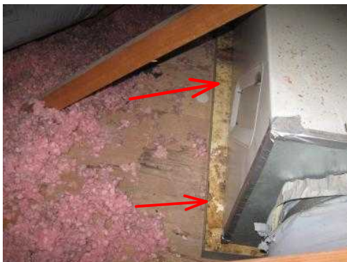
Refer to seller for disclosure. There is rusting noted in the overflow pan under the heating unit in the attic. Refer to seller disclosure. Consult a licensed HVAC contractor for evaluation and
