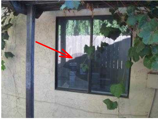
Cracked/broken window noted at right/front bedroom ; repair, as required.
