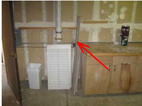
GFCI protection required at all added garage outlets. Safety Hazard.
