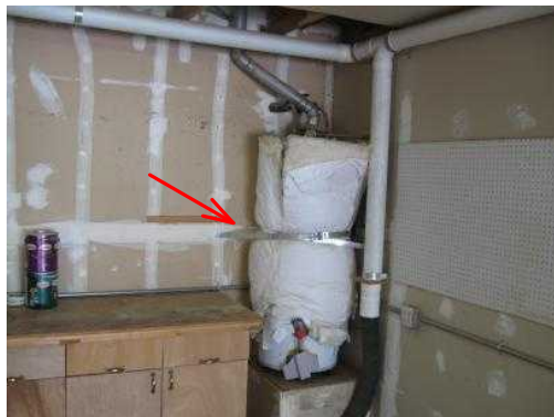
Water heater earthquake (seismic restraint) support straps missing or not properly installed.
