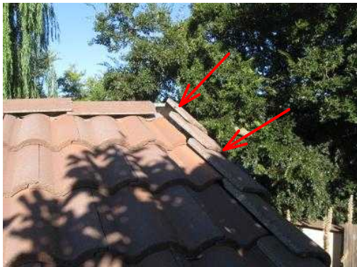
Loose front ridge and edge caps noted, above the garage. Repair, as required.
