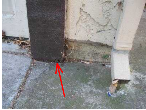
Wood deterioration noted to the trim, at right base of right/front roll-up garage door.
