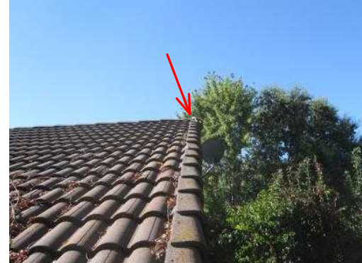
Left and right side end area ridge caps are missing/loose. Repair, as required.
