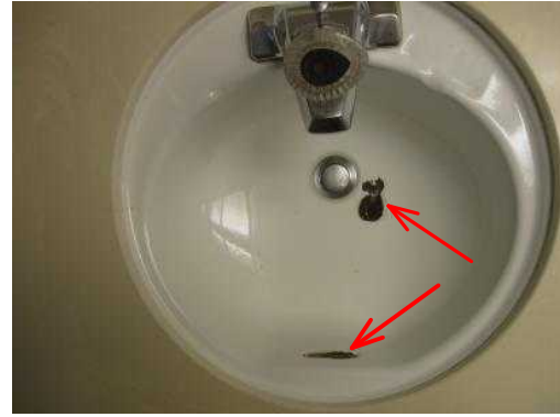
Rusting at the overflow drains and on the underside of master bathroom sinks.
