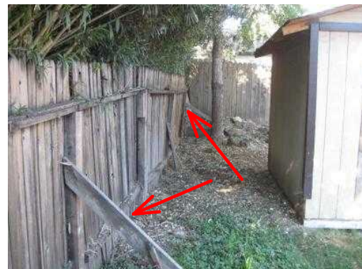
Rear fence sections are being held up by boards. Right/rear fence section is broken/damaged.
