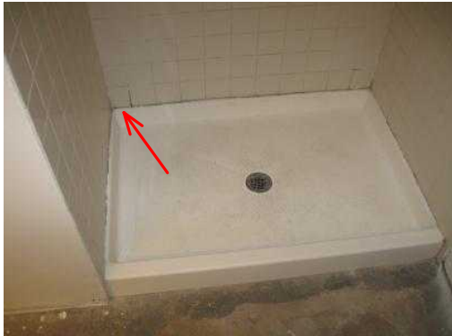
Grout needs work, at the bottom courses of master shower tile; repair, as required.
