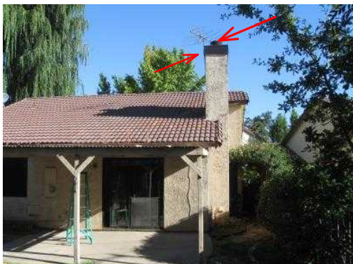
Chimney has a cap and spark arrester. Antenna is mounted to chimney, causing unnecessary stress.
