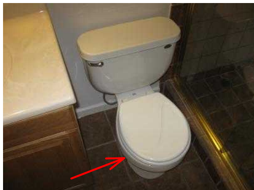
The hall bathroom toilet is loose at the floor and will require replacement of the wax seal.
