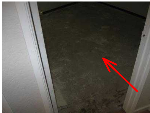
Missing right/middle bedroom area flooring. Cracking noted at the slab.
