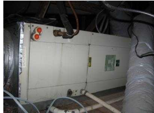
Shows view of the heating unit heat pump in the attic space. Original unit is 24 years old.
